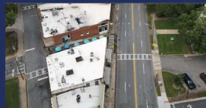
Before four to three lane conversion
